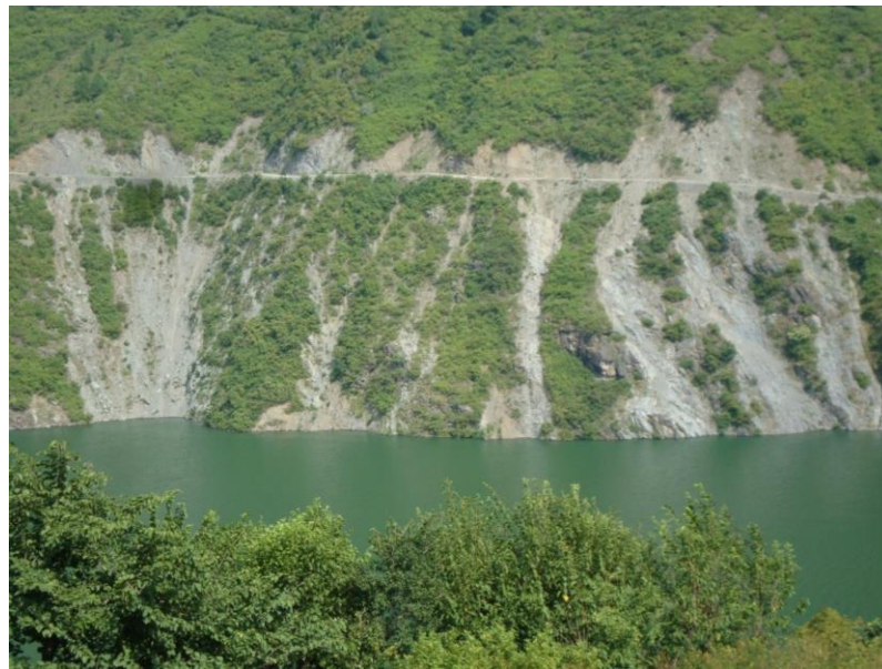
Fig. 1.1 Some landslides were detected along the reservoir embankment in the Tehri region.
