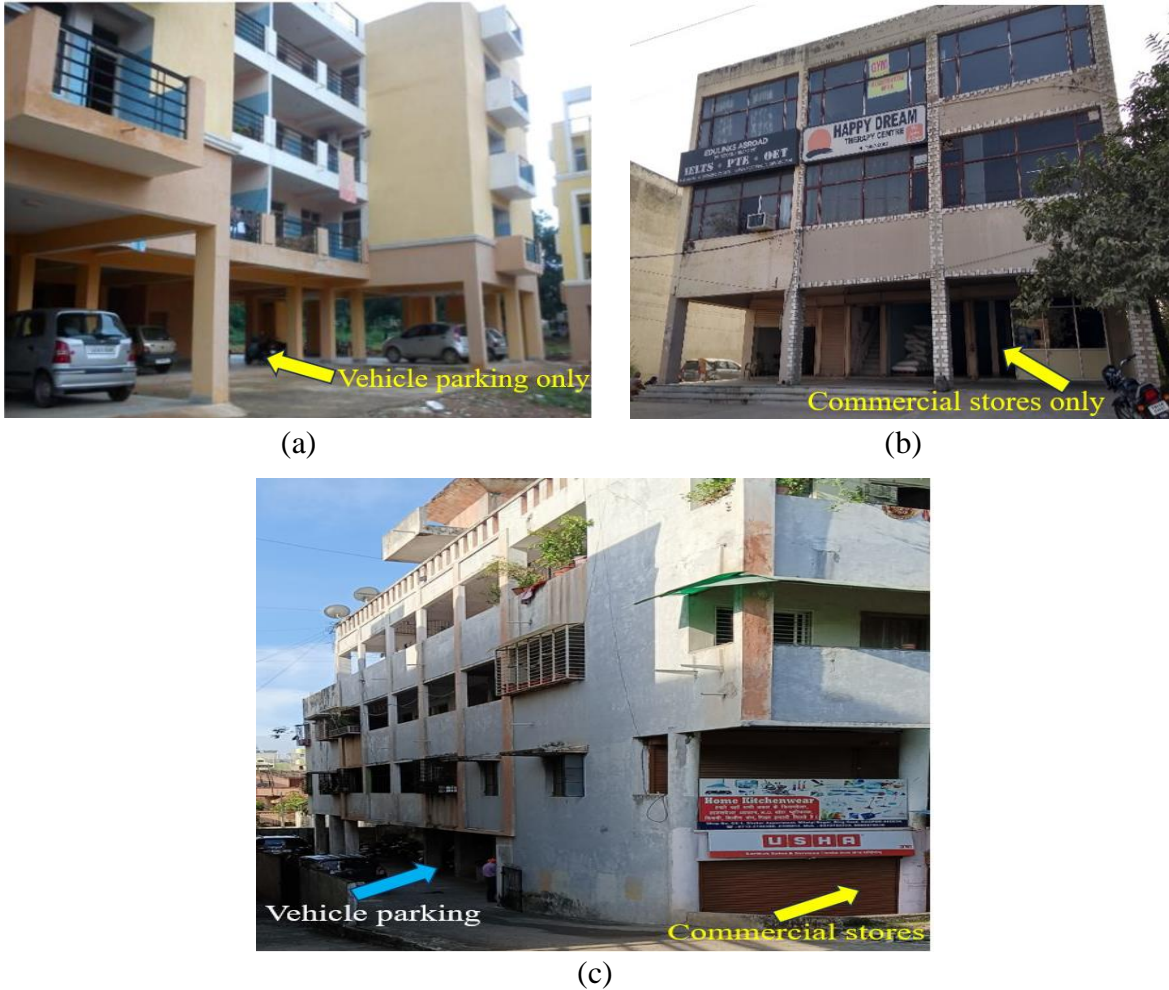
Fig. 6.1 Typical RC buildings with irregular placement of infills to serve the purpose of (a) vehicle parking only; (b) commercial stores only; and (c) combination of both vehicle parking and commercial stores at the ground storey while upper storey(s) used for residential purpose
