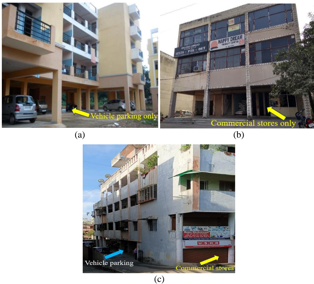
Fig. 1.1 Typical RC buildings with irregular placement of infills to serve the purpose of (a) vehicle parking only; (b) commercial stores only; and (c) combination of both vehicle parking and commercial stores at the ground storey while upper storey(s) used for residential purpose
