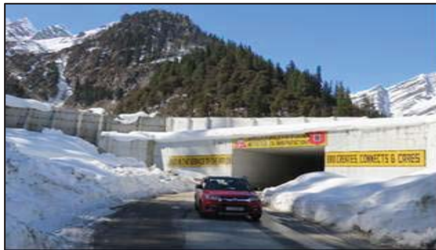
Figure 1.13: A 120 m long snow shed at MSP-7 avalanche site, Dhundhi, H.P., India
