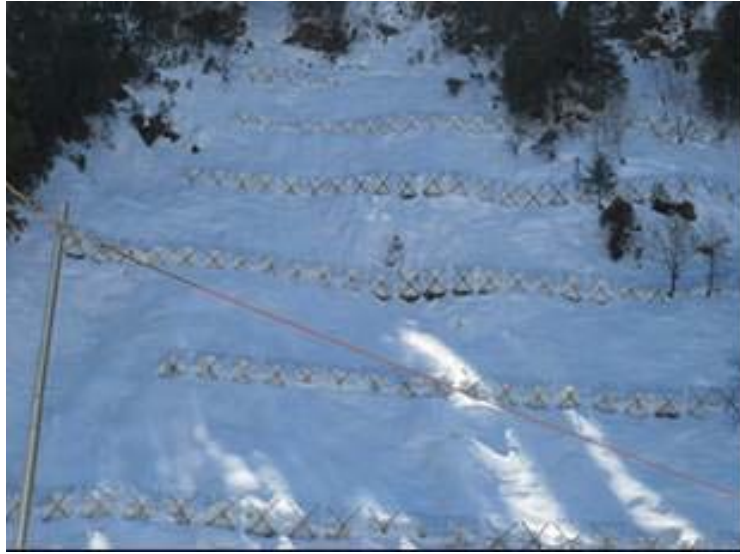
Figure 1.11: Snow umbrella type structures installed in the formation zone at MSP-6 site, Dhundhi, Himachal Pradesh, India
