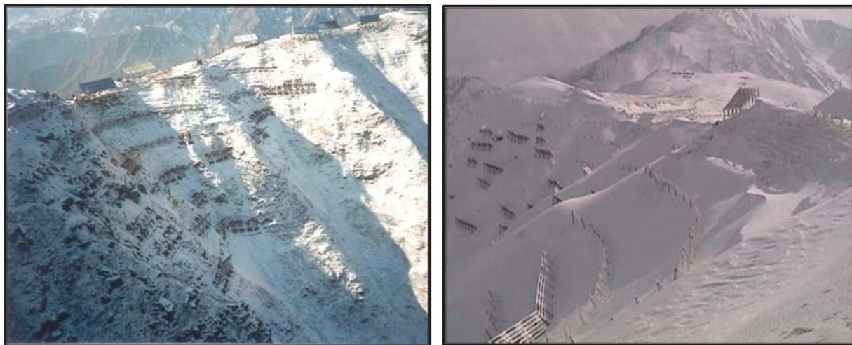
Figure 1.10: Snow bridge structures in the formation zone at Banihal top, J & K, India
