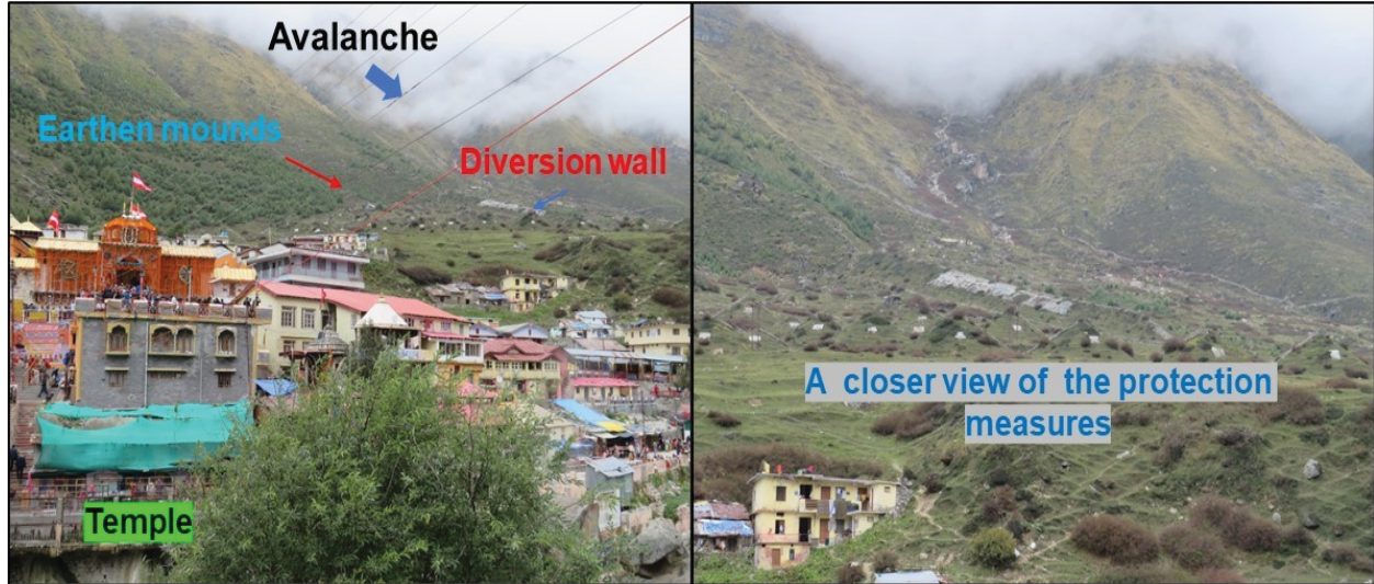
Figure 1.15: Integrated scheme of earthen mounds and diversion wall used for the protection of Shri Badrinath temple, Uttarakhand, India
