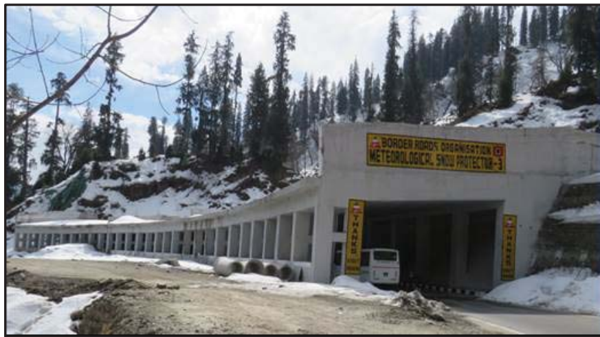
Figure 1.12: A 135 m long snow shed at MSP-3 avalanche site, Dhundhi, H.P., India
