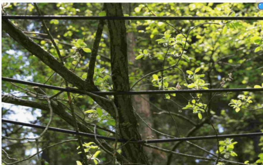
Figure 2.3 Example of a high-impedance fault occurs when tree branches come into contact with overhead CCs [26].
